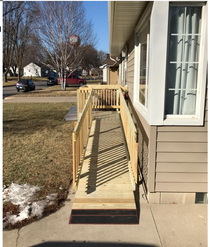
Wooden modular ramp with landing next to house.
